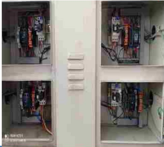
ON & OFF Timers arranged for IBT Agitators
